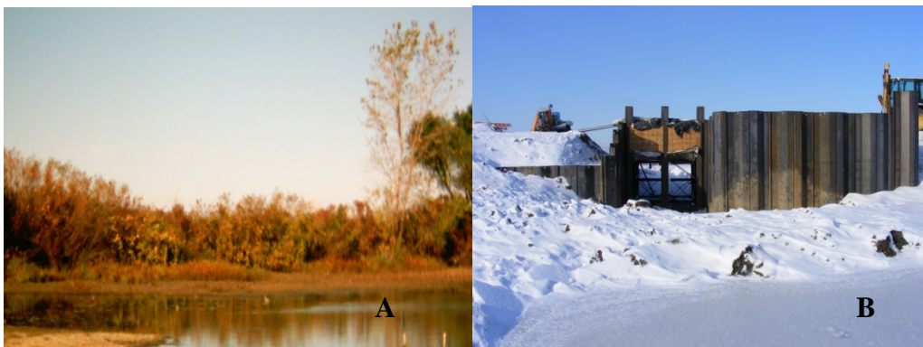
Figure 1. A) Pre-Construction at site B) Progress on water-control structure as of Dec. 15, 2010
