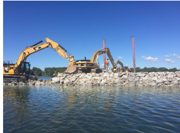
Figure 2. Shoal construction operation.
